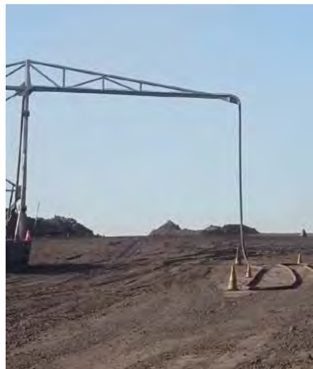
Cable suspended above guideways
